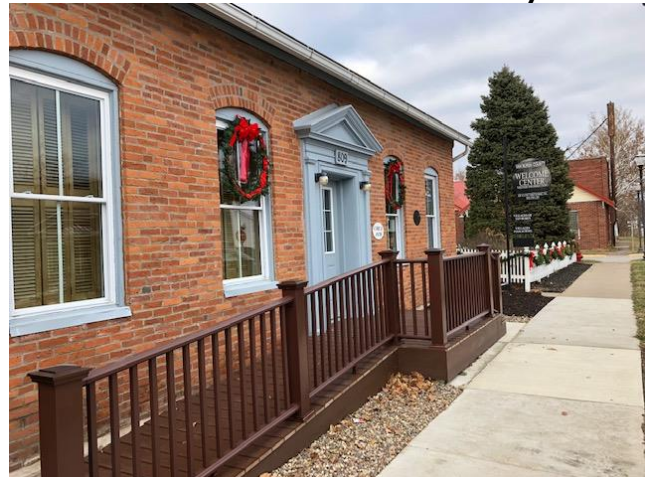
Ramp makes the Welcome Center accessible to all.
